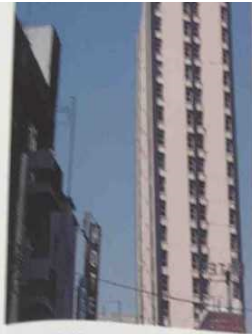
Figure 11.12 The building on the left is in the process of falling over during an earthquake in Mexico. The sediment underneath it is acting like quicksand.
