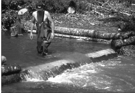
Digger Log being placed in a stream
