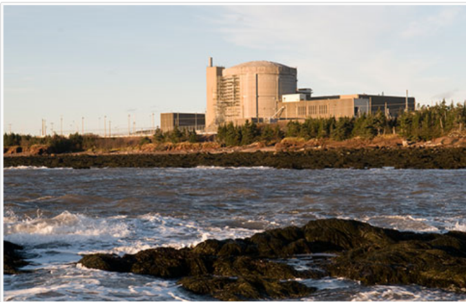
View of the Point Lepreau Generating Station
